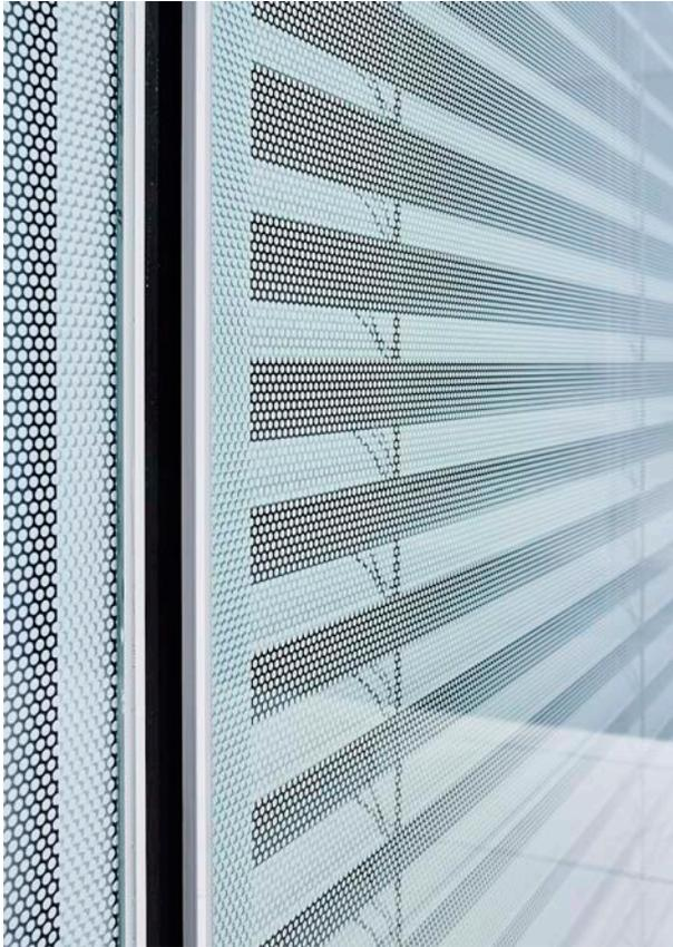
If necessary, the solar radiation can be regulated with a Venetian blind behind the baffle pane, which is printed with a dot screen.
