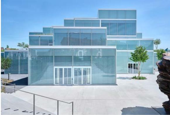
The outward appearance of the SQUARE is distinguished by the exposed concrete framework and closed double-skin façade.
