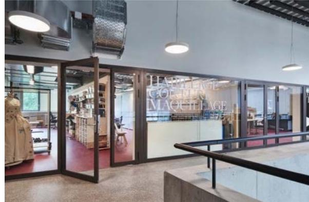
*Transparency and fire protection in the foyers and corridors are ensured by glass partitions and doors with Forster fuego light E130 as well as fixed glazing and fire-retardant doors with Forster presto E30. Photos: © Damian Poffet*
