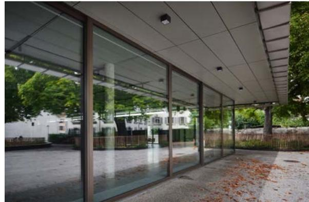
*An aesthetic and technical link between the existing building and the new construction. The doors and fixed glazing were realised with the Forster unico steel profile system, both in the theatre building (left in the photo on the left) and in the adjacent function hall. Photos: © Damian Poffet*
