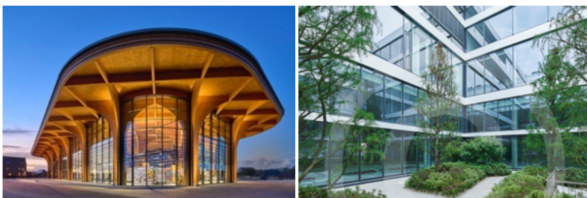
Thermally insulated curtain walls with fire protection: The forster thermfix vario profile system is based on a mullion/transom construction. With its slim face widths of just 45 millimetres, it allows for a wide range of large-scale applications. Photos: © Ronald Tilleman (left), © Damian Poffet (right)
