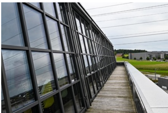
The forster thermfix vario Hi steel profiles, which are only 45 millimetres wide, provide passive-house-level heat insulation in the sloping facade on the top floor. Photos: Huber Kontech AG
