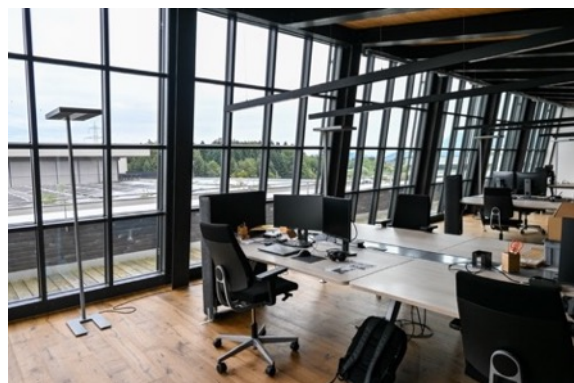
The forster thermfix vario Hi steel profiles, which are only 45 millimetres wide, provide passive-house-level heat insulation in the sloping facade on the top floor. Photos: Huber Kontech AG
