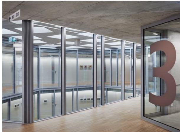
*The corridors lead around the building in a closed circuit and offer residents intuitive orientation, while the generous glazing towards the atrium with forster thermfix vario EI60 ensures maximum daylight on the floors. Photos: © Damian Poffet*
