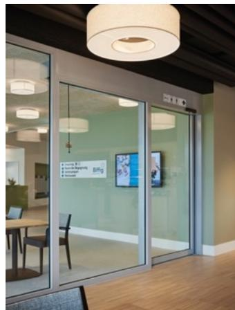
*The restaurant on the ground floor has safe, barrier-free access thanks to the automatic fire protection sliding door with forster fuego light EI30. Photos: © Damian Poffet*
