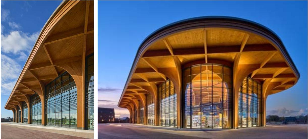
*In order to ensure the exceptional sustainability and long service life of the SuperHub, the architectural designers chose the forster thermfix vario energy-efficient facade system for thermally insulated curtain walls that offer Passive House-standard thermal insulation. The curved facade of the building features double glazing. Photos: © Ronald Tilleman*
